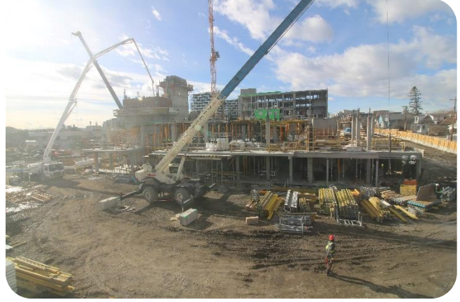
Mobile cranes on site. Formwork for columns main to second floor and second floor slab being installed.
