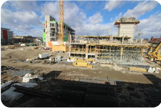
East tower concrete is complete and exterior framing in progress. Elevator shaft walls almost complete.
